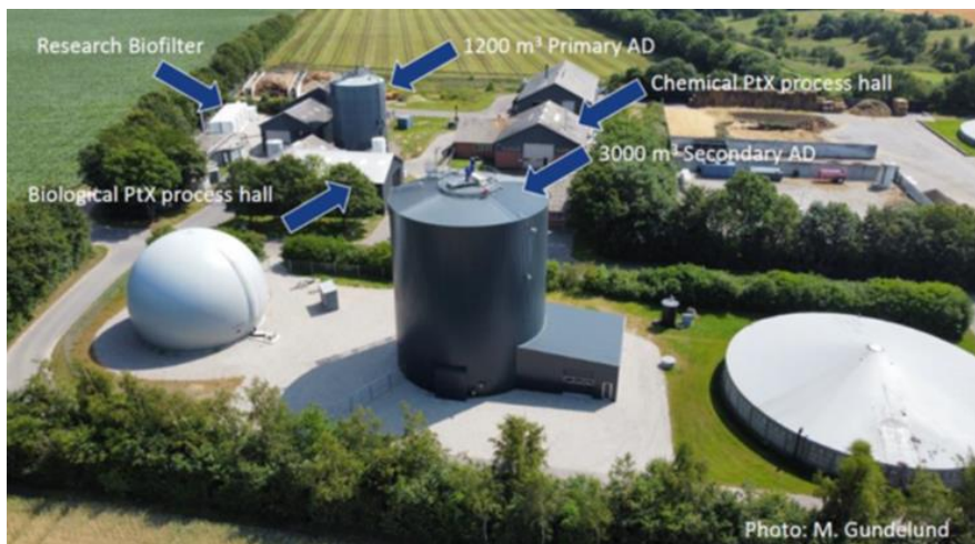
Figure 34: Aarhus University Biogas and Power-to-X facility located at AU Campus Viborg.
