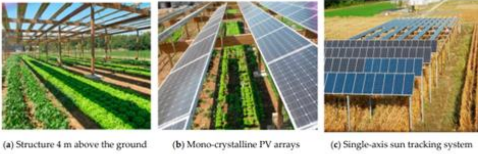
Figure 3. Experimental agrivoltaic system in Montpellier, France. © C. Dupraz.
