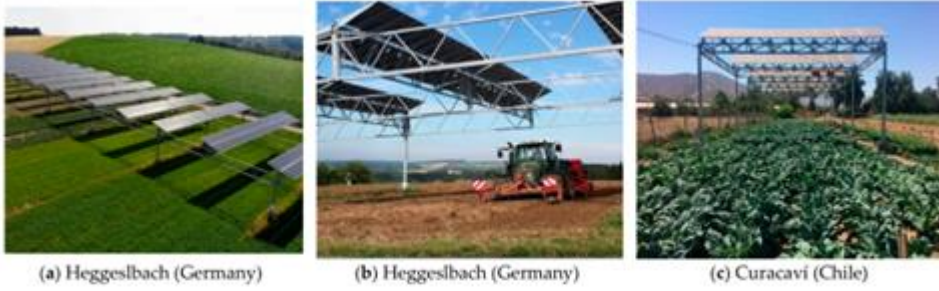
Figure 4. Experimental agrivoltaic systems installed by Fraunhofer ISE in Germany (a,b) and Chile (c). © Fraunhofer ISE.
